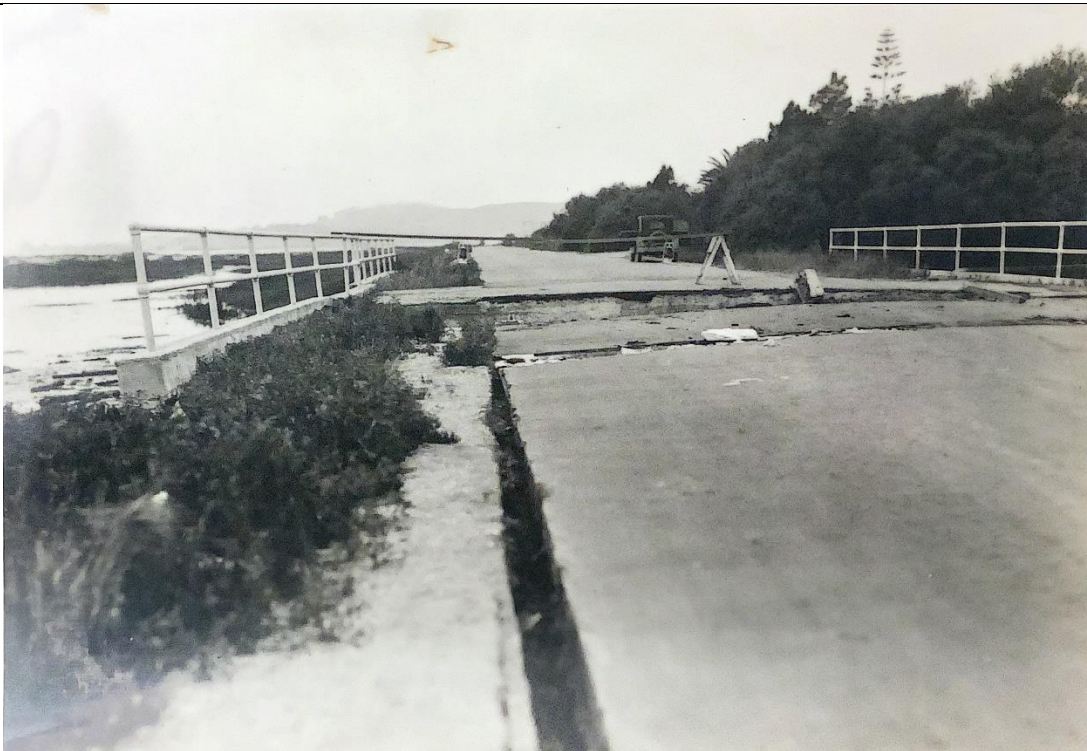
Figure 30. Displaced road on the Boulevard along the beach as the result of subsidence. The road is offset one to two feet. Photo credit: Santa Barbara Historical Museum, Gledhill Library.
