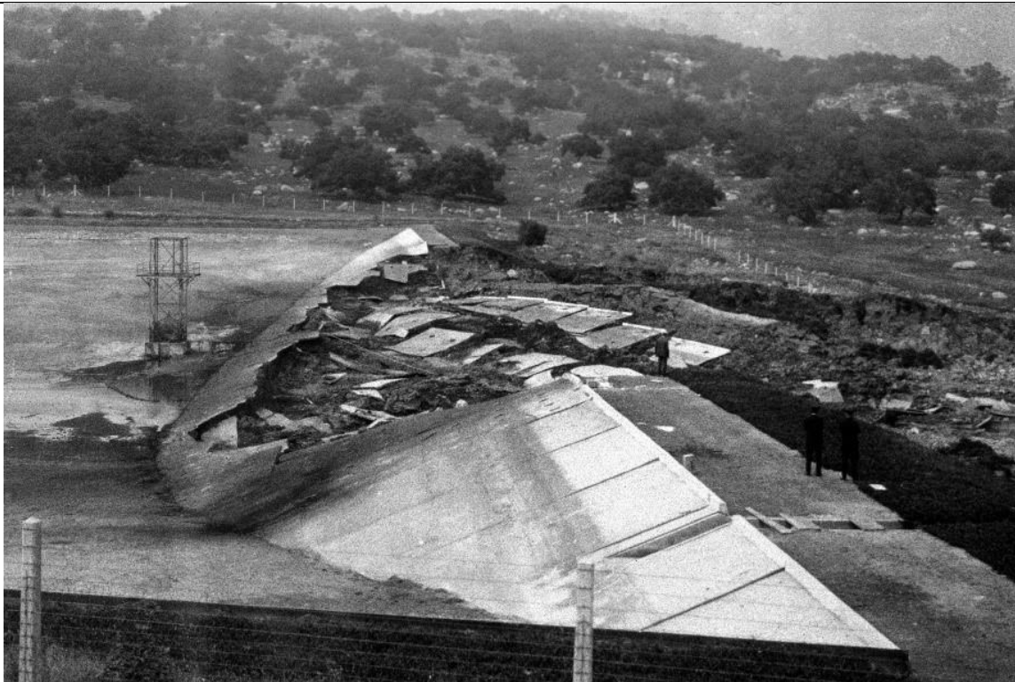
Figure 33. Close up view of the dam after the landslide failure of the earthen dam. Photo credit: California Department of Dam Safety Archives in Association of State Dam Safety Officials.
