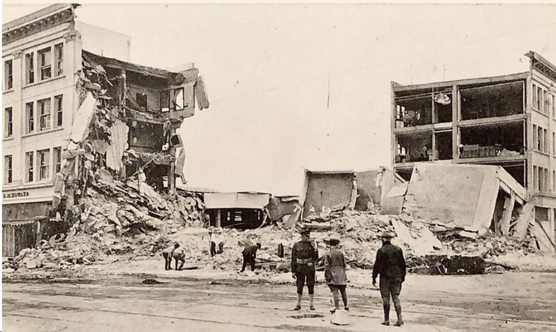
Figure 13. Postcard photographs of before and after the earthquake of the four-story San Marcos Building. Sylvester and Mendes (2001) note that the building was constructed in several sections that were not structurally tied together, and they suggest that battering of the two wings occurred during the shaking. Two people were killed in the collapse of the building. Only one wing of the building was rebuilt and it is now a two-story building. The San Marcos building is located on the southeast corner of State Street and Anapamu Street. Photo credit: Santa Barbara Historical Museum, Gledhill Library.
