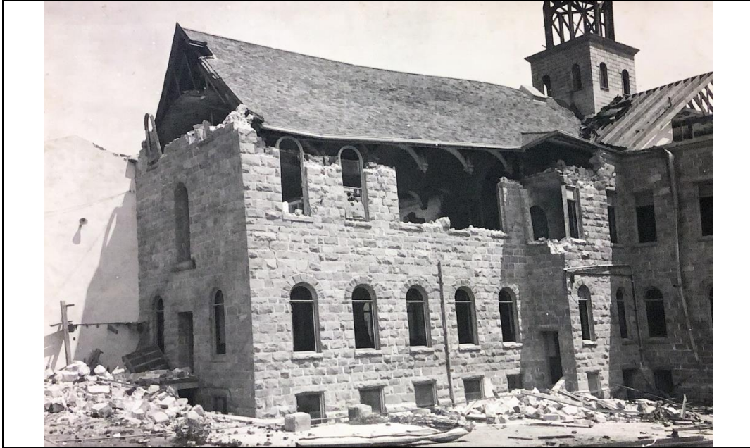
Figure 24. The sandstone masonry of St. Anthony's Seminary was damaged, and portions of the wall collapsed. Photo credit: Santa Barbara Historical Museum, Gledhill Library.
