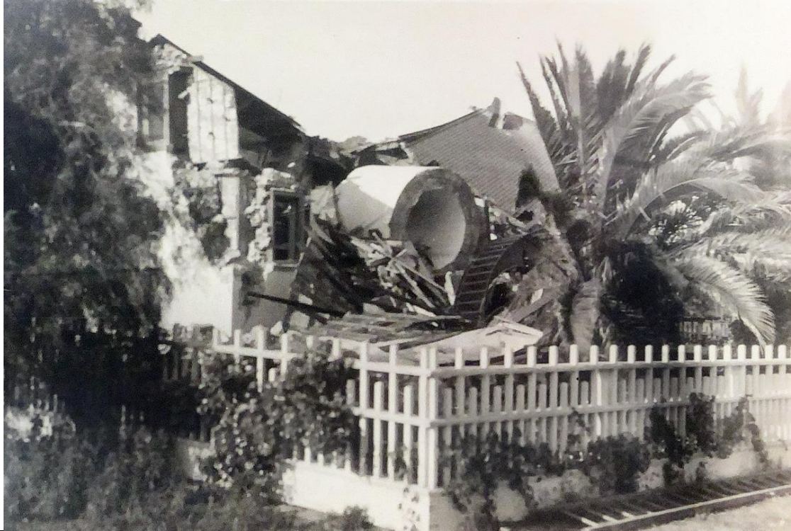
Figure 20. View of the collapsed lighthouse tower that crushed the home of the light keeper. Photo credit: Santa Barbara Historical Museum, Gledhill Library.
