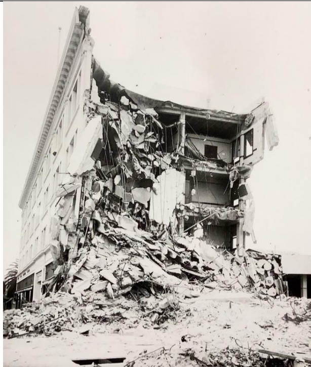
Figure 15. View of the destruction of the east wing of the San Marcos Building. State Street is on the left side of the building. Photo credit: Santa Barbara Historical Museum, Gledhill Library.
