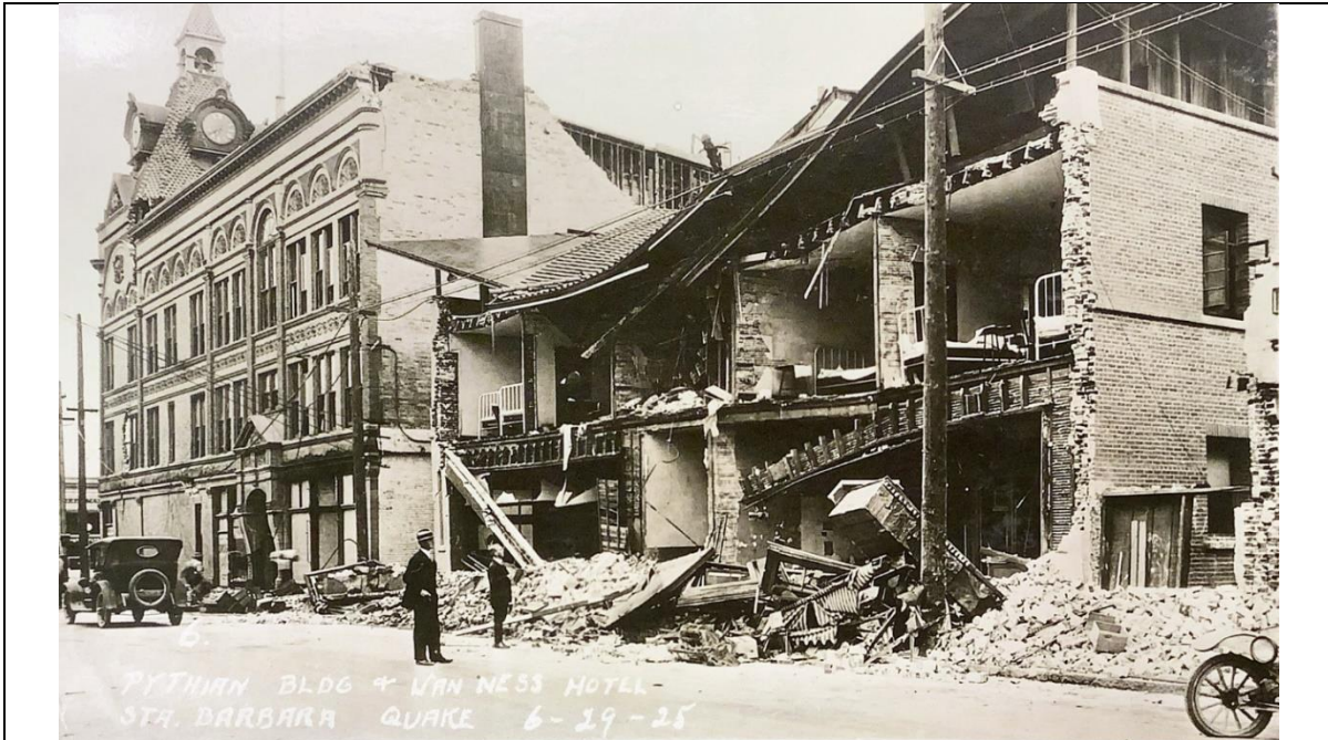
Figure 12. The Van Ness Hotel with a collapsed wall and roof sits next to the Fithian Building. The brick masonry wall of the Fithian Building in the upper center of the photograph has collapsed. Photo credit: Santa Barbara Historical Museum, Gledhill Library.
