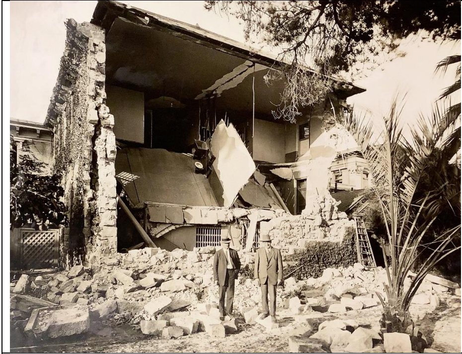
Figure 16. The unreinforced stone masonry structure of the County jail was severely damaged. Standing in front was Supervisor Sam Stanwood (left) and Sheriff Jim Ross (right). Note the collapsed second story floor inside the structure. Photo credit: Santa Barbara Historical Museum, Gledhill Library.
