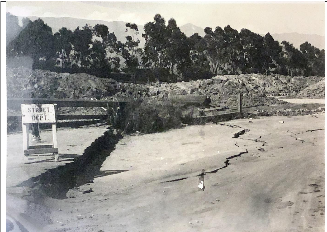
Figure 31. Displaced and tilted road surface produced by subsidence in Santa Barbara, however the specific location is unknown. Photo credit: Santa Barbara Historical Museum, Gledhill Library.
