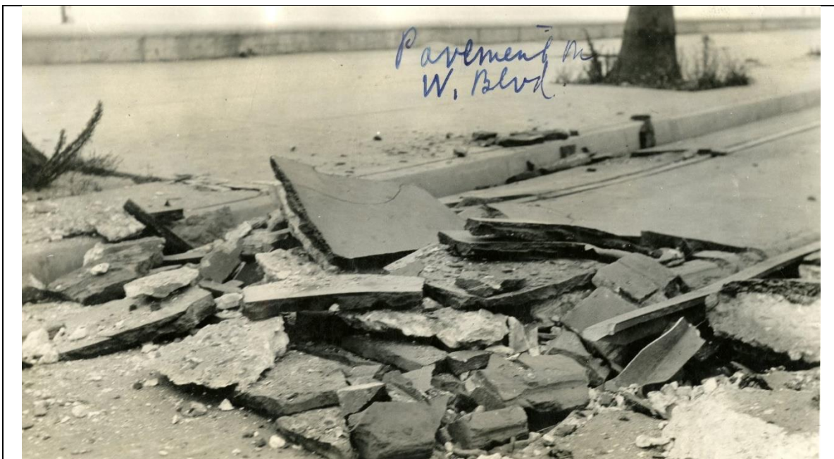
Figure 27. Broken pavement and trolley tracks on West Cabrillo Boulevard. Minor buckling of the gutter along the southeastern side of the road can be seen in the upper right of the photograph. Photo credit: Courtesy of the Edson Smith Photo Collection, Santa Barbara Public Library.
