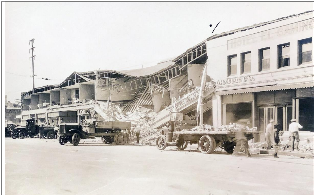
Figure 11. Auto row was destroyed by the earthquake as seen in the photograph where the partial collapse of second story lodging fell in the auto showrooms below. Photo credit: Santa Barbara Historical Museum, Gledhill Library.
