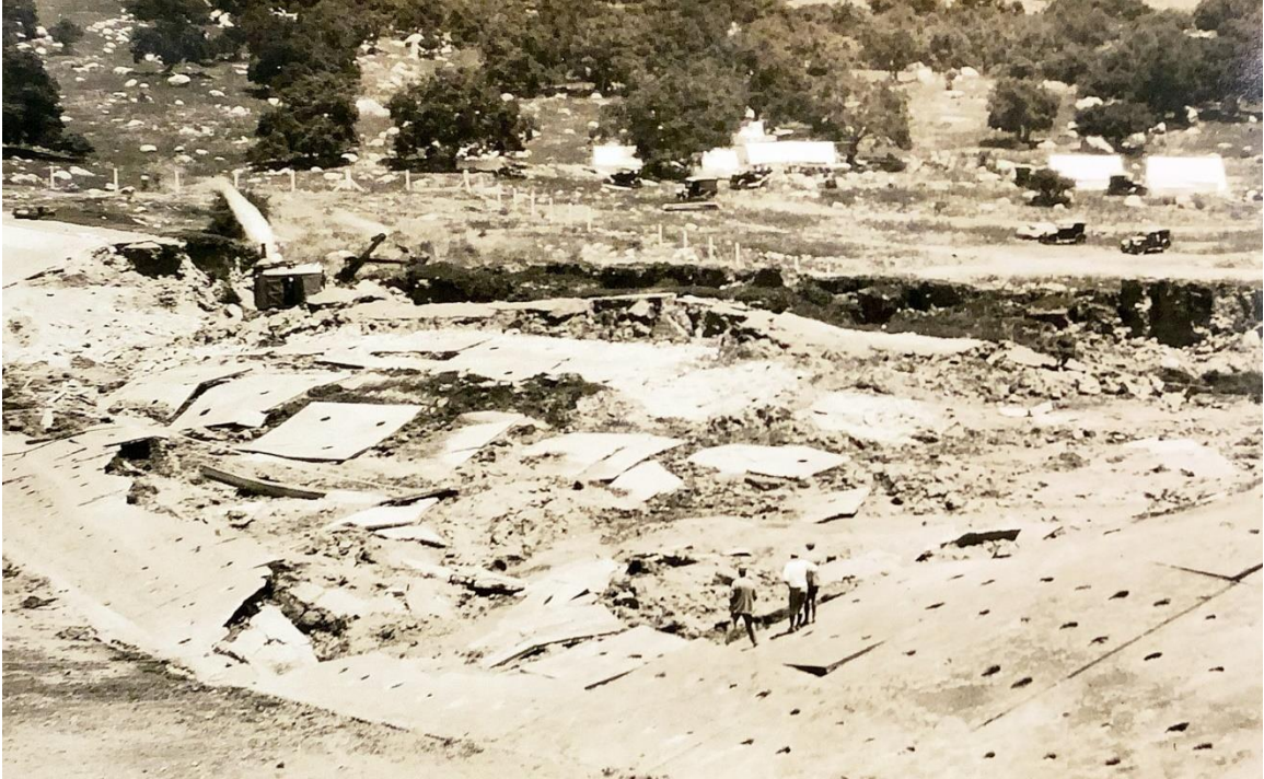
Figure 34. Wide angle perspective looking at the drained reservoir (left of dam) and the landslide formed on the earthen dam. Photo credit: California Department of Dam Safety Archives in Association of State Dam Safety Officials.
